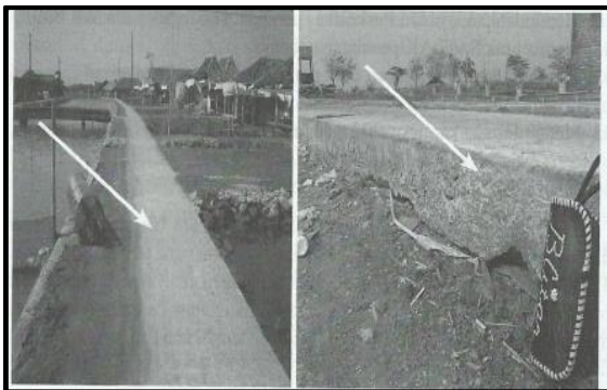
Figure 14. Raising the public road
