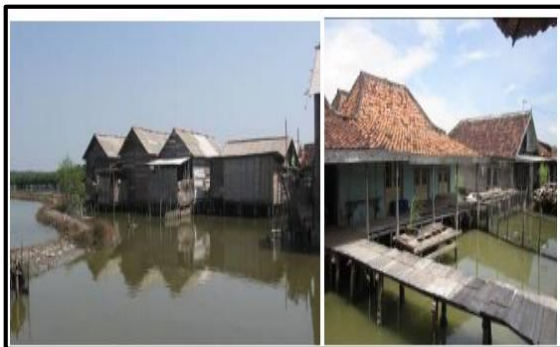
Figure 13. Establishing House on Stilts for New House
