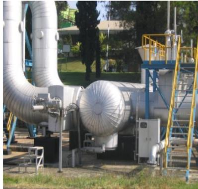
**Gambar 3.4** *Steam Receiving Header*
