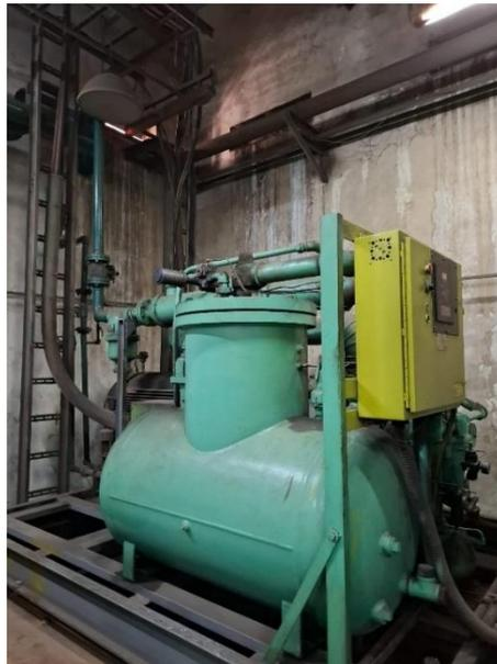
**Gambar 4.1** *Compressor Screw* Unit 5-7
