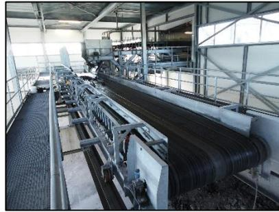
**Gambar 3. 11** *Conveyor Bottom Ash Power Plant*
