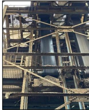
**Gambar 4.4** *Conveyor 16 Unit 5 mengalami Mistracking*
