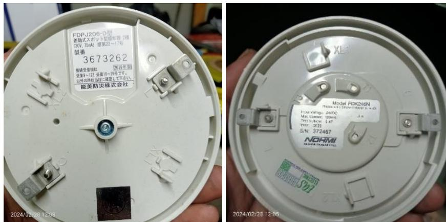
**Gambar 4.1** *Heat Detector Dan Smoke Detector*
