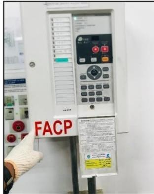
**Gambar 3.7** *Fire Alarm Control Panel*
