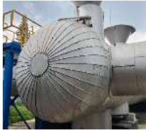
**Gambar 3.4** *Steam Receiving Header*
