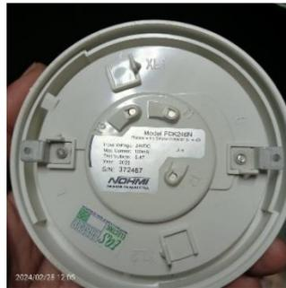
**Gambar 4. 1** *Fire alarm Type Smoke*
