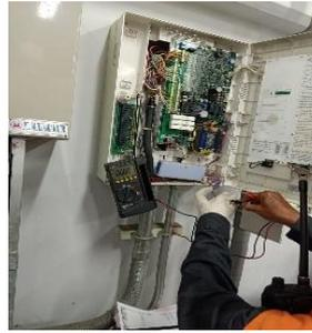
**Gambar 3. 5** FACP(Fire alarm Control Panel)
