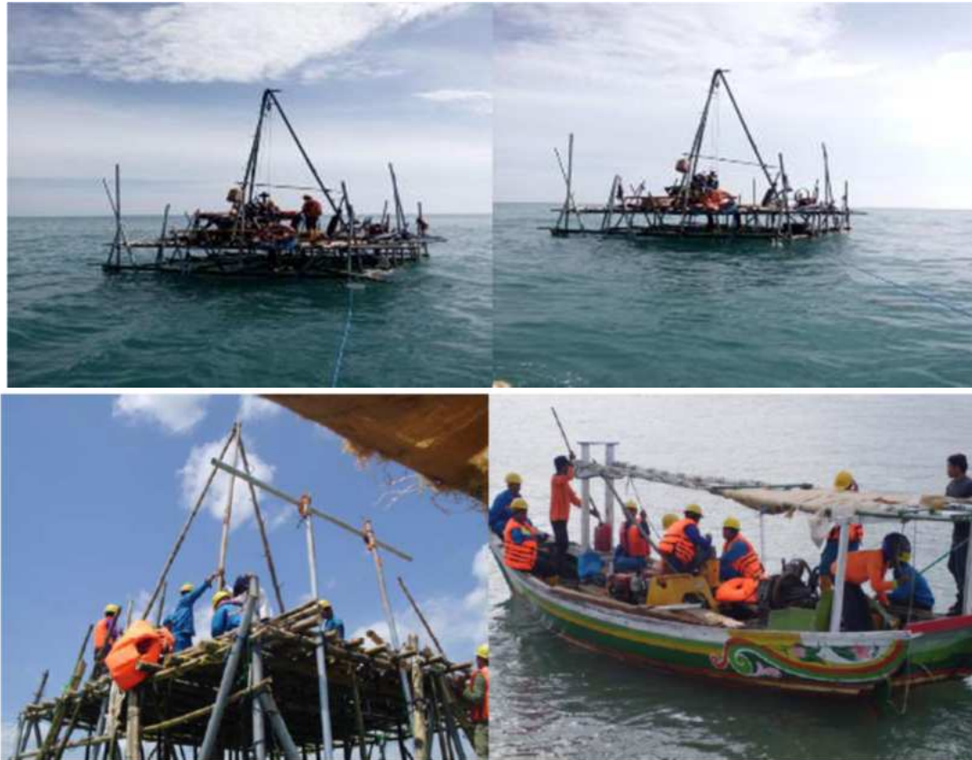
Figure 2-2 Moving Rig to Platform
