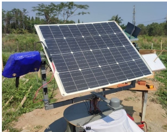
Gambar 4.3 Kondisi panel surya kegelapan shading 0%
