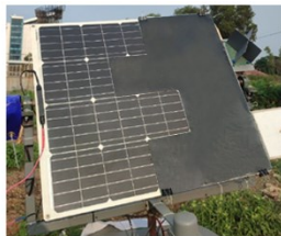
(b) Penutupan 1/2 panel
