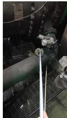
**Gambar 4.11** *Cleaning valve dan pipa backwash debris*
