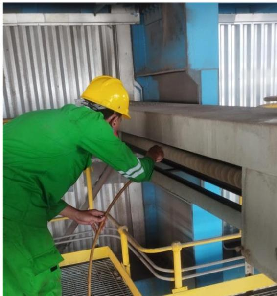
**Gambar 4.6** Pembersihan *Track Beam Rail*
