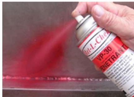
Gambar 2.6 Penetrant Test (pipingengineer.org)
