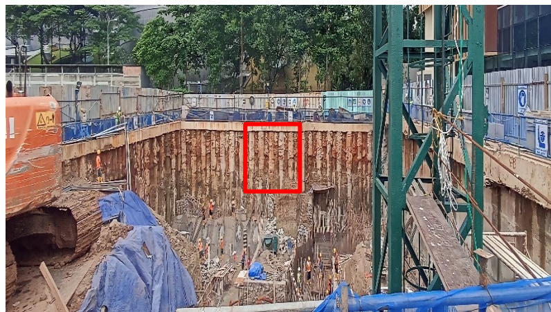
Gambar 4.4 Titik Contiguous Bored Pile
