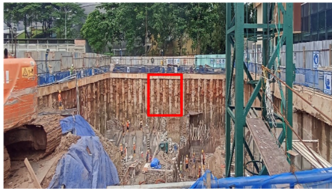
Gambar 4.4 Titik Contiguous Bored Pile
