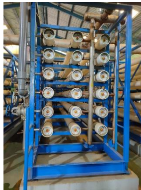
Gambar B.2 Unit Membran Reverse osmosis
