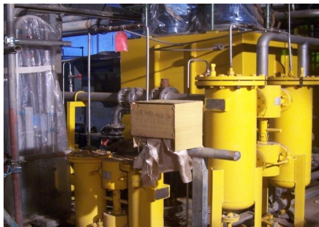
Gambar 3.1. BFPT lube oil system
