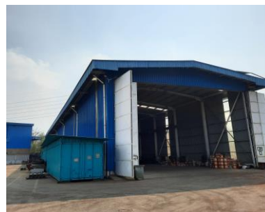
Gambar 2.6 Blasting & Painting Shop
