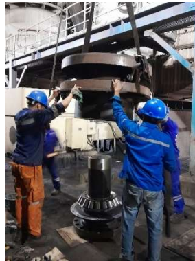
Gambar 4.7 Masukkan Housing Bearing (Sumber: Dokumen Pribadi)
