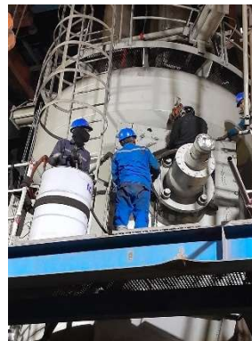
Gambar 4.9 Grinding Roller Terpasang
