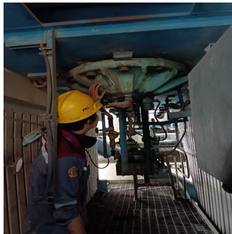
Gambar 5. 6 Pengecekan Support Bearing
