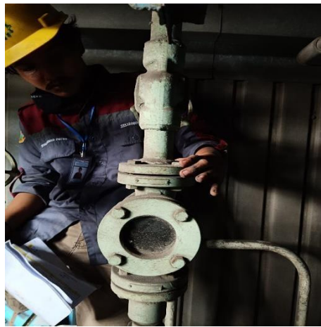
Gambar 5. 4 Pengecekan Pompa Pendingin Oli Support Bearing
