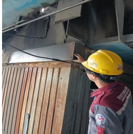
Gambar 5. 5 Pengecekan Expansion Joint
