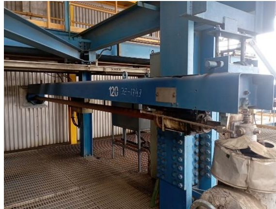
Gambar 4.2 Long Retractable Sootblower
