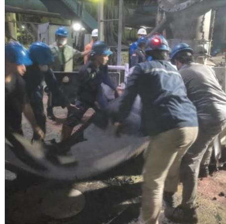
2. *CM Pyrite Guide Mill Pulverizer Pergantian Seal Piston*
