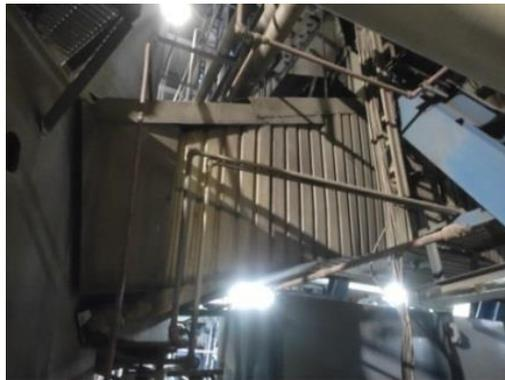
**Gambar 4.12** Memeriksa Kebocoran *Pressure Air Duct*
