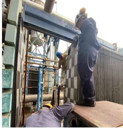
Gambar 4.7 Pemasangan Plate Heat Exchanger (Sumber : Pribadi)
