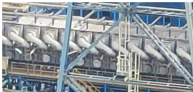
Gambar 3.5 Desalination Supply Pump (Sumber : Dokumen Pribadi)
