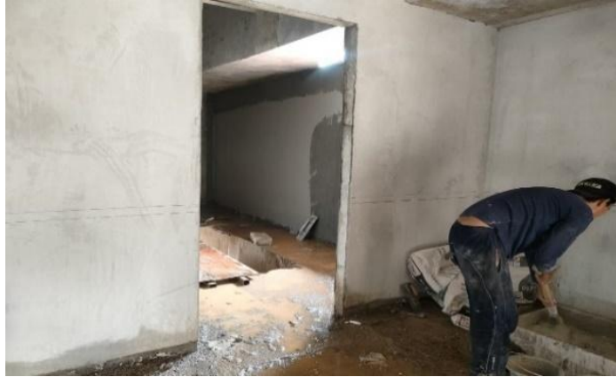
Gambar 3.25 Acian Dinding Lantai 2 Gereja SPMBG
