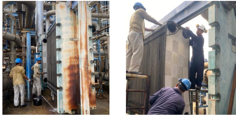
Gambar 4.3 Proses Pembersihan & Pengecekan Plate
