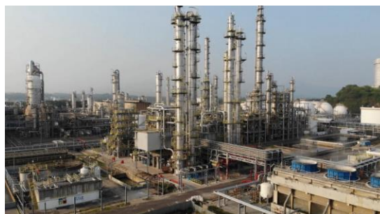
Gambar 2.9 MTBE & B1 Plant
