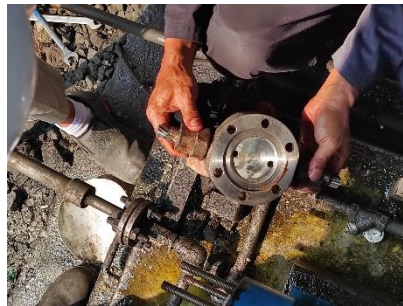
Gambar 4.6 Pengecekan dan pembersihan head Pump
