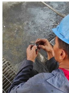
Gambar 4.9 Proses Inspeksi Bolt Oil Drain
