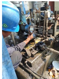
Gambar 4.10 Memasang Bolt Oil Drain
