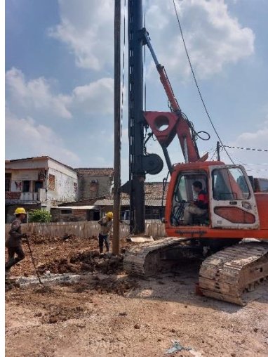
Gambar 4.1 Drilling Machine Bore Pile
