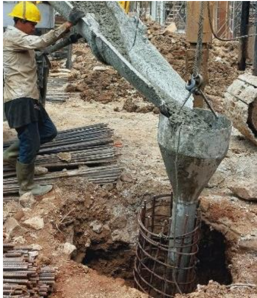
Gambar 4.40 Proses Pengecoran Bore Pile
