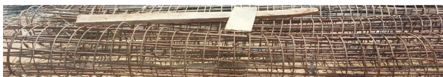
Gambar 4.22 Besi Bore Pile
