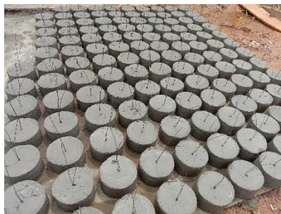
Gambar 4.18 Beton Decking
