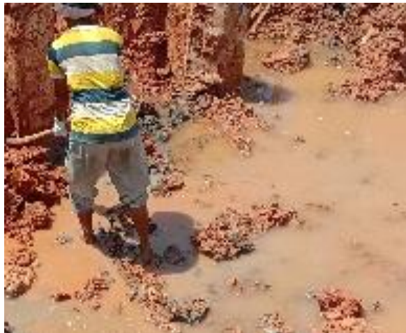
Gambar 4.42 Proses Galian Pile Cap
