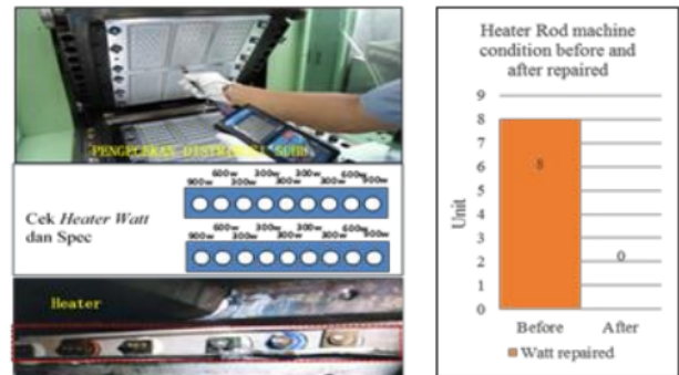
Figure 5: Repairing All Rod Heater Machines
