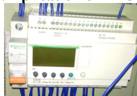
Figure 2. PLC (Smart Relay Zelio) [8]
